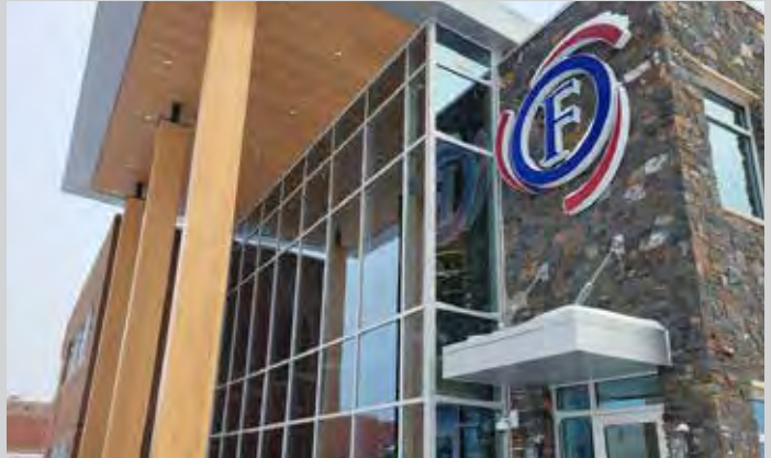
Exterior of Park Falls building located at 177 4th Ave. S.
